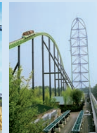
ACCELERATOR: KINGDA KA T.H.C.: 1400 pph Height: 138 m (456 ft) Track length: 940 m (3109 ft) No. of trains: 4x18 pers.
