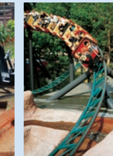
MINE TRAIN COASTER T.H.C.: 860 pph Height: 17 m (56 ft) Track length: 517 m (1696 ft) No. of trains: 1 x 26 pers.
