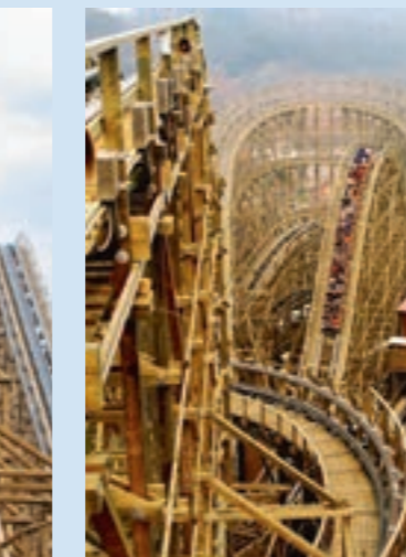
WOODEN COASTER T.H.C.: 1500 pph Height: 44 m (144 ft) Track length: 1655 m (5430 ft) New track technology
