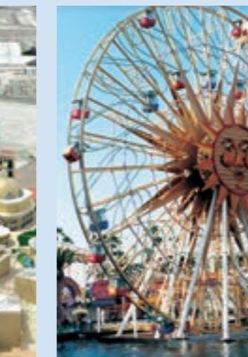
COASTER WHEEL T.H.C.: 1000 pph Height: 48 m (157 ft) No. of gondolas: mobile 16, fixed 8 Capacity per gondola: 6 pers.
