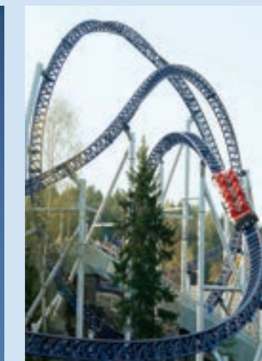
ACCELERATOR WITH INVERSIONS T.H.C.: 740 pph Height: 32 m (105 ft) Track length: 690 m (2264 ft) No. of trains: 2x12 pers.
