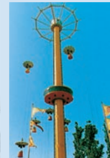
PARACHUTE GYRO TOWER T.H.C.: 1920/3120 pph Cabin capacity: 70 No. of parachutes: 12 Height: 83.5 m (274 ft)
