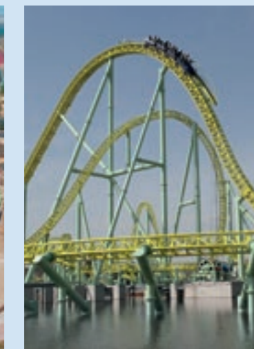
MEGA-LITE COASTER T.H.C.: 820 pph Height under: 40 m (131 ft) Track length: 755 m (2477 ft) No. of trains: 2x16 pers.
