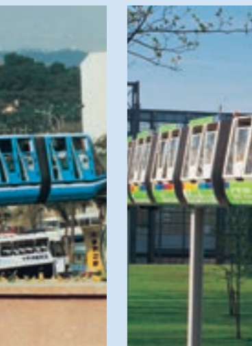
MONORAIL P6/60 Gelsenkirchen, Germany T.H.C.: 3000 pph No. of trains: 11 Track length: 2500 m (8202 ft)
