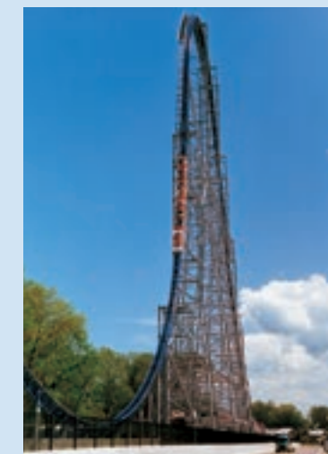
GIGA COASTER T.H.C.: 1650 pph Height from: 80 m (263 ft) Track length from: 2000 m (6560 ft) No. of trains: 2-3x36 pers.
