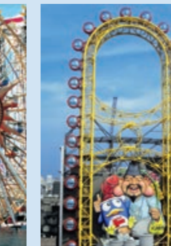
GIANT WHEEL ON BUILDING T.H.C.: 640 pph Height: 78 m (246 ft) Number of gondolas: 32 Capacity per gondola: 4 pers.
